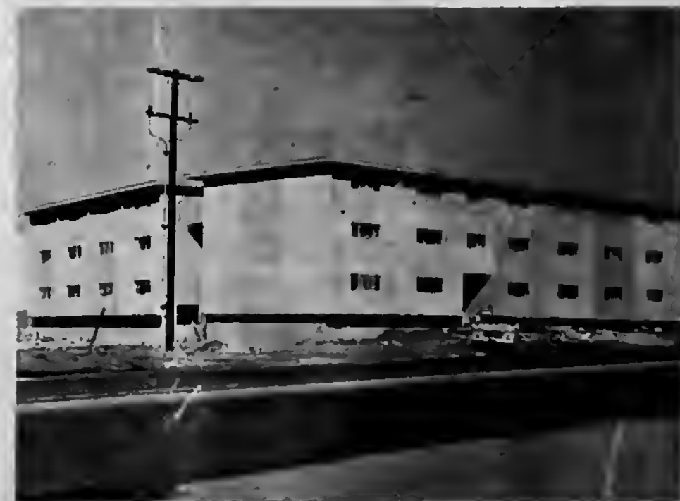
New McAfee Apartments NEAR completion.
